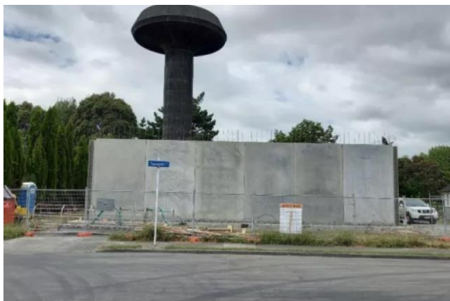
Figure 14: New Bulls Reservoir near the old water tower.
