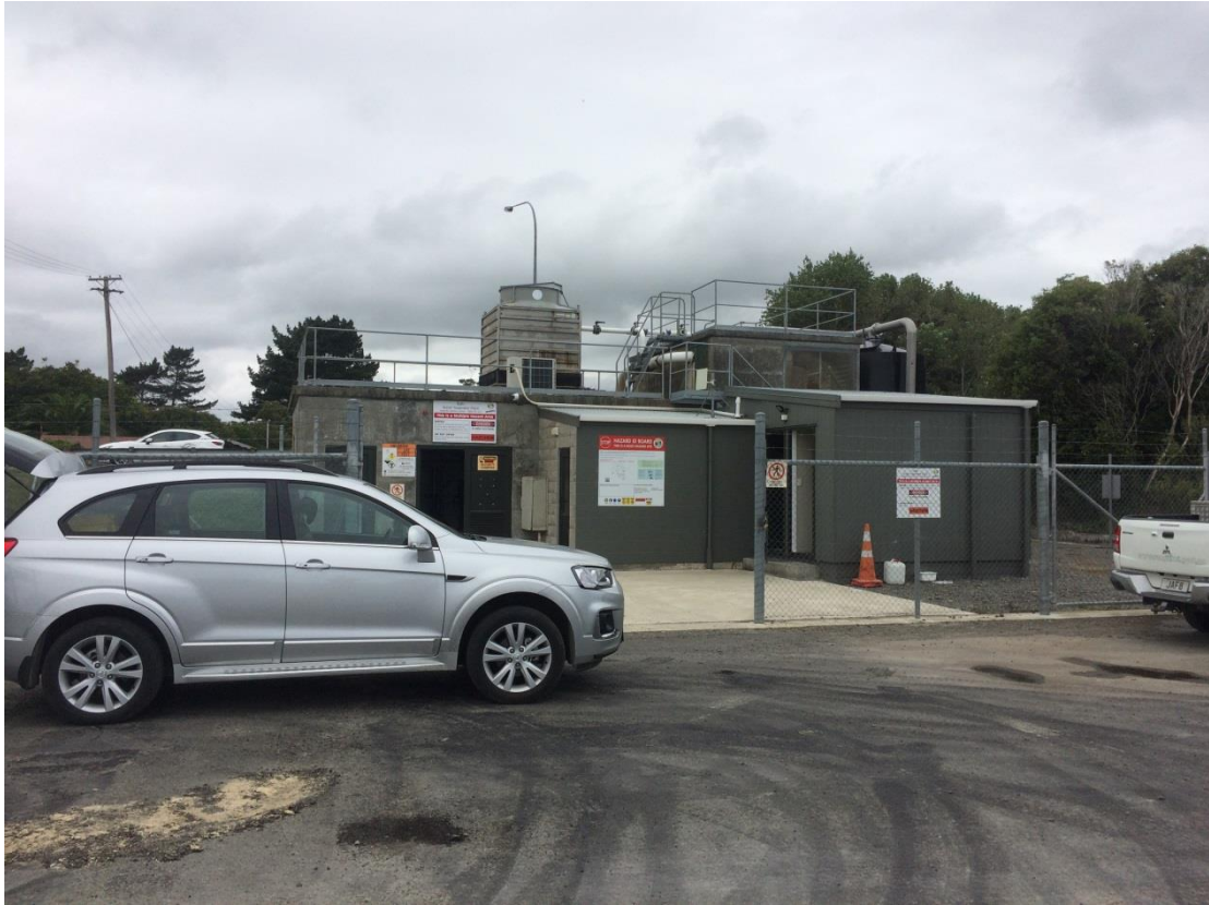
Photograph 1: Bulls Water Treatment Plant
