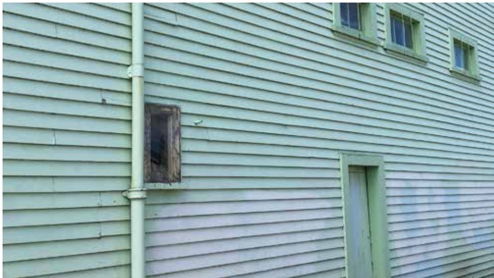
Original weatherboard cladding
