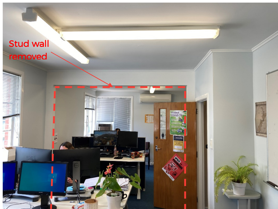
Figure 4: Office with new Gib lining and internal wall removed
