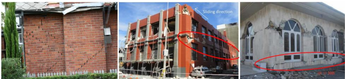
Figure 2. In-Plane Failures of URM Wall (NZSEE Guidelines)
