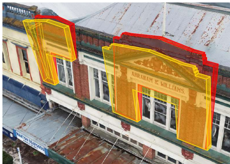
Figure 12. Local failure mechanism analysis for Abraham and Williams' front façade
