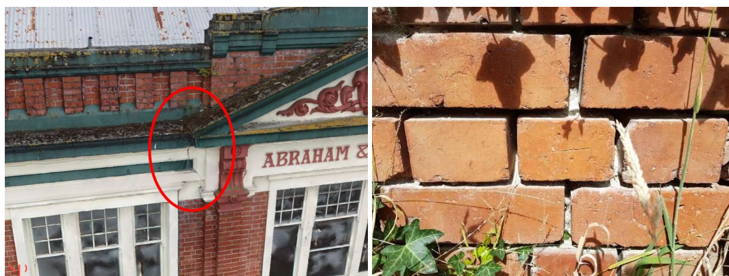
Figure 6. Cracks in Abraham and Williams façade and washed out mortar joints
