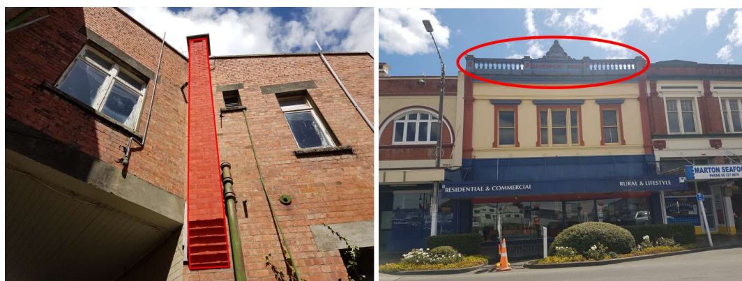
Figure 7. Protruding URM chimneys that extend pass the roofline and heavy ornaments/parapets at the top of Davenport's façade
