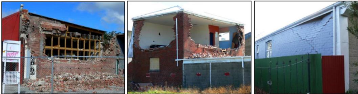
Figure 1. OOP Failure of URM Wall (BRANZ)
