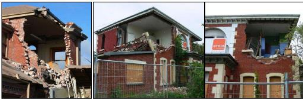
Figure 4. Examples of Building Corner Failures (BRANZ)
