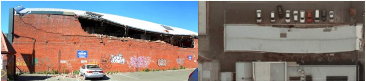
Figure 3. OOP Failure due to Diaphragm Displacement (NZSEE Guidelines)
