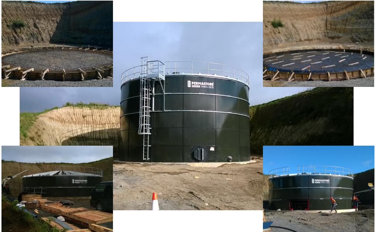
Above: Construction of the 766m 3 green glass coated steel tank.
