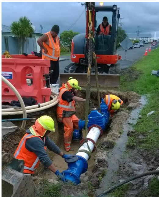
Above: Installing valves and fire hydrants on Kaitere Street.
