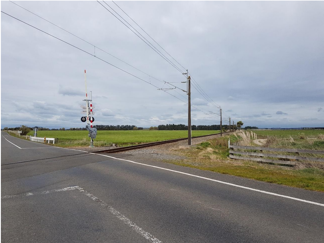
Figure 12: West Approach – looking south from 1.5m back from limit line
