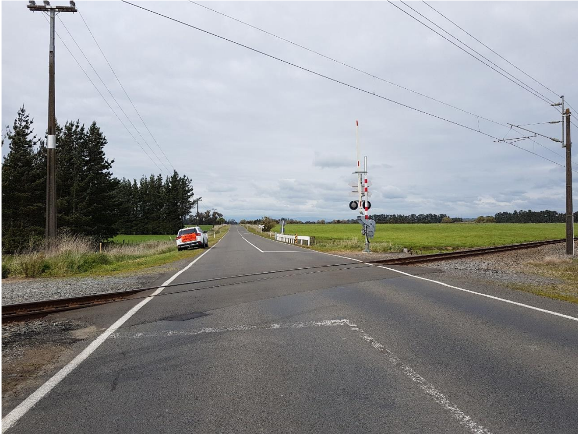
Figure 13: West Approach – looking east from 1.5m back from limit line
