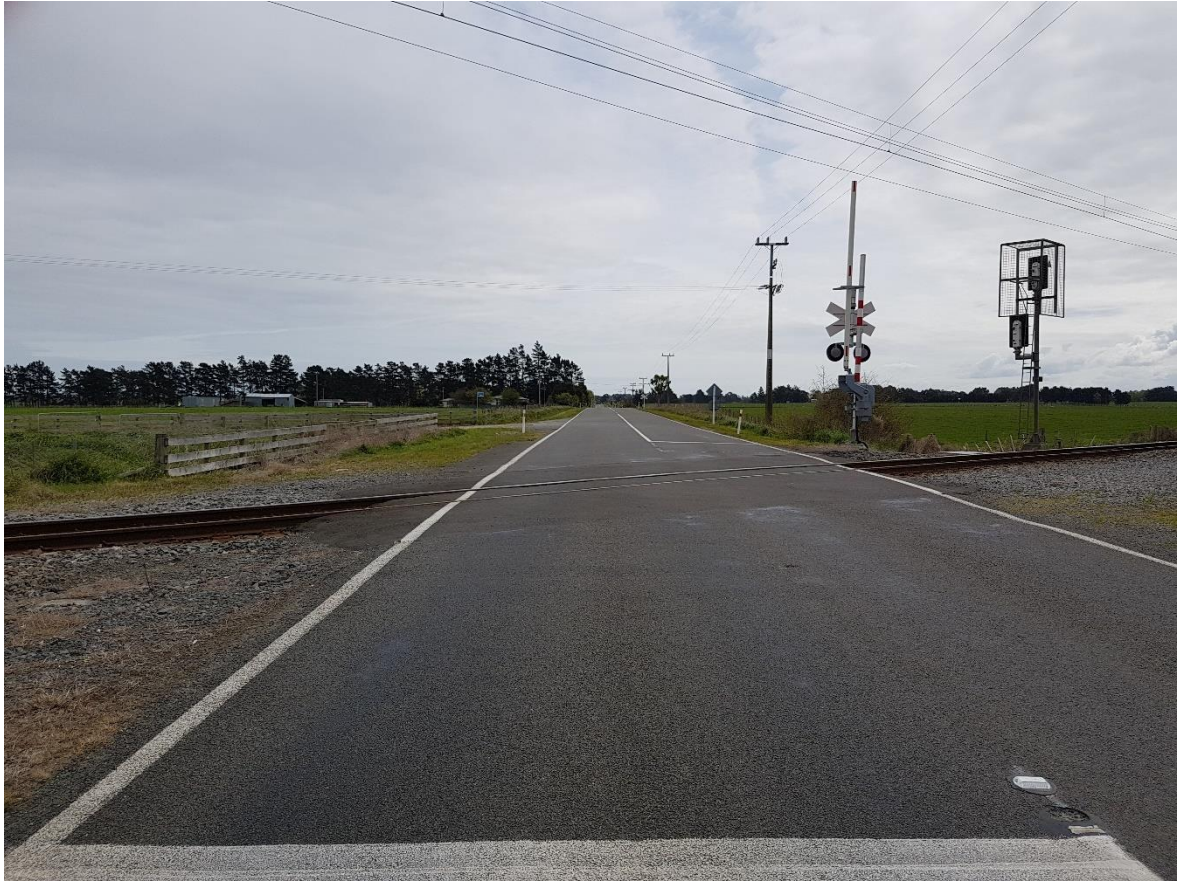
Figure 7: East Approach – looking west from 1.5m back from limit line
