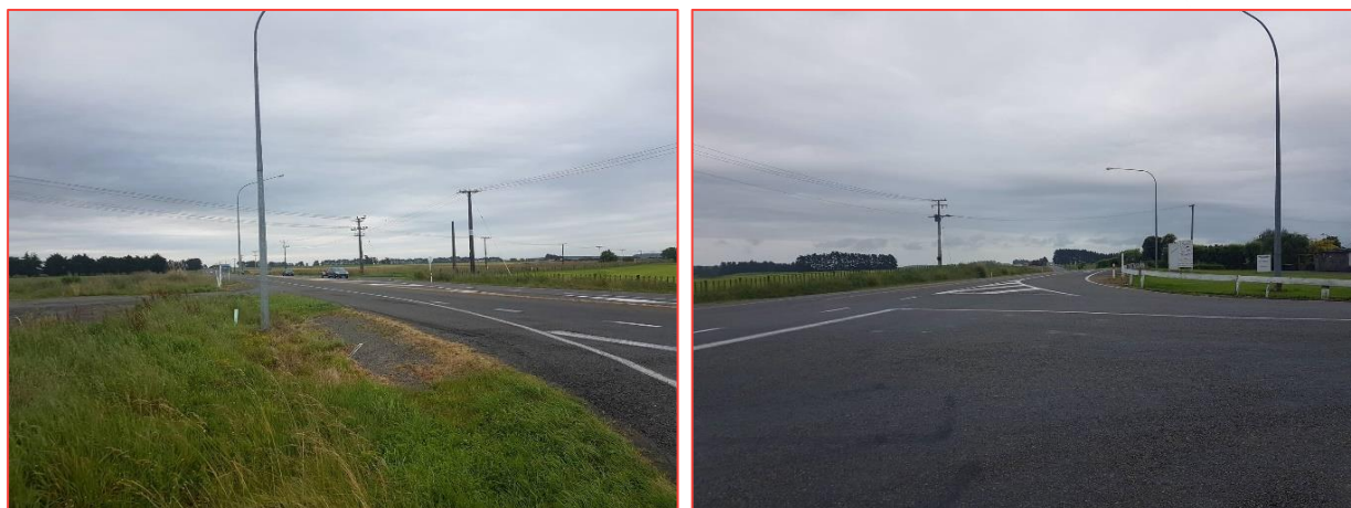
Figure 4-15: View at the Pukepapa Road / SH3 Intersection to the East (Left) and West (Right)
