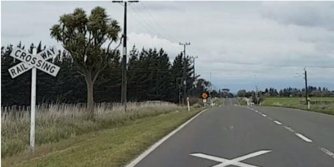
Figure 10: West Approach Makirikiri Road – looking east from 100m west of crossing
