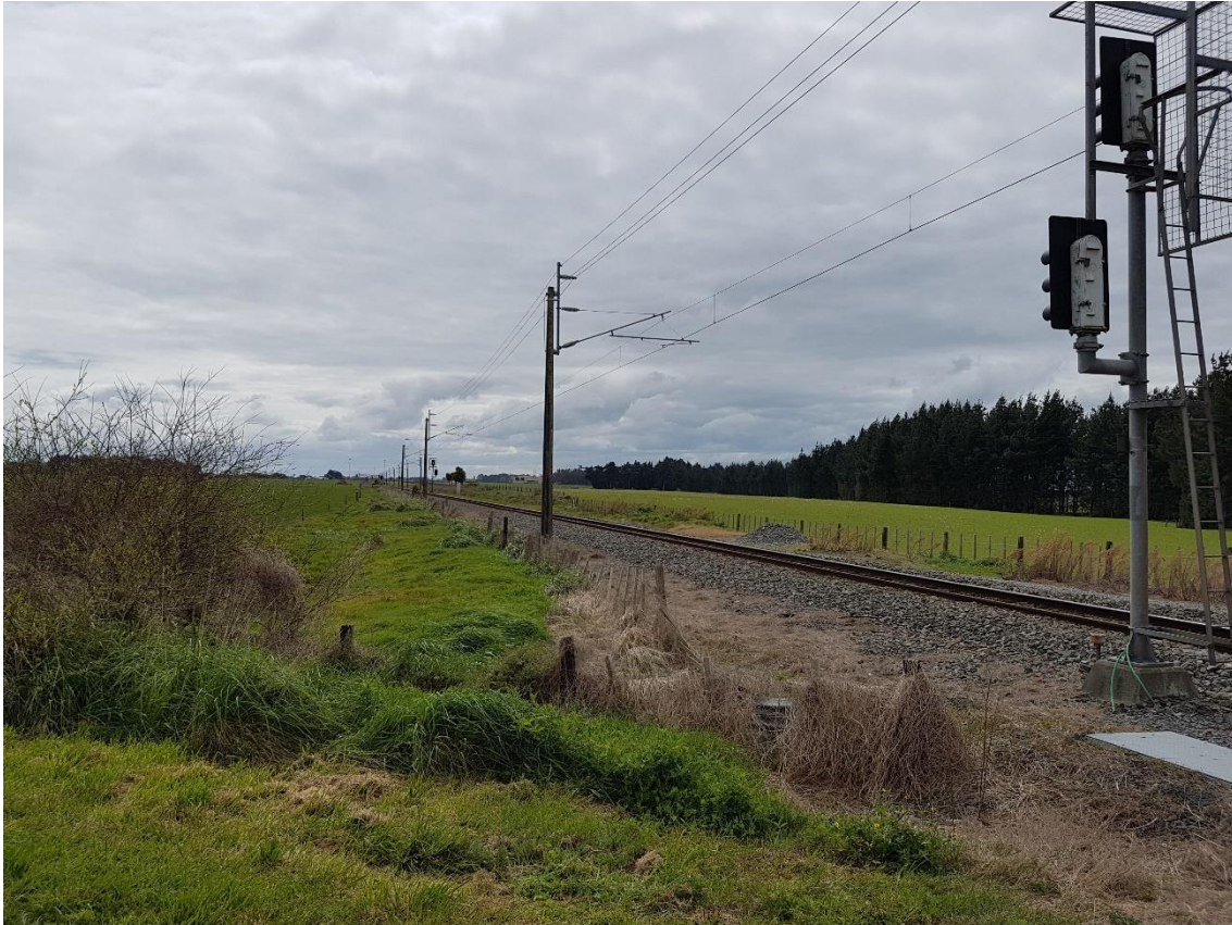
Figure 11: West Approach – looking north from 1.5m back from limit line
