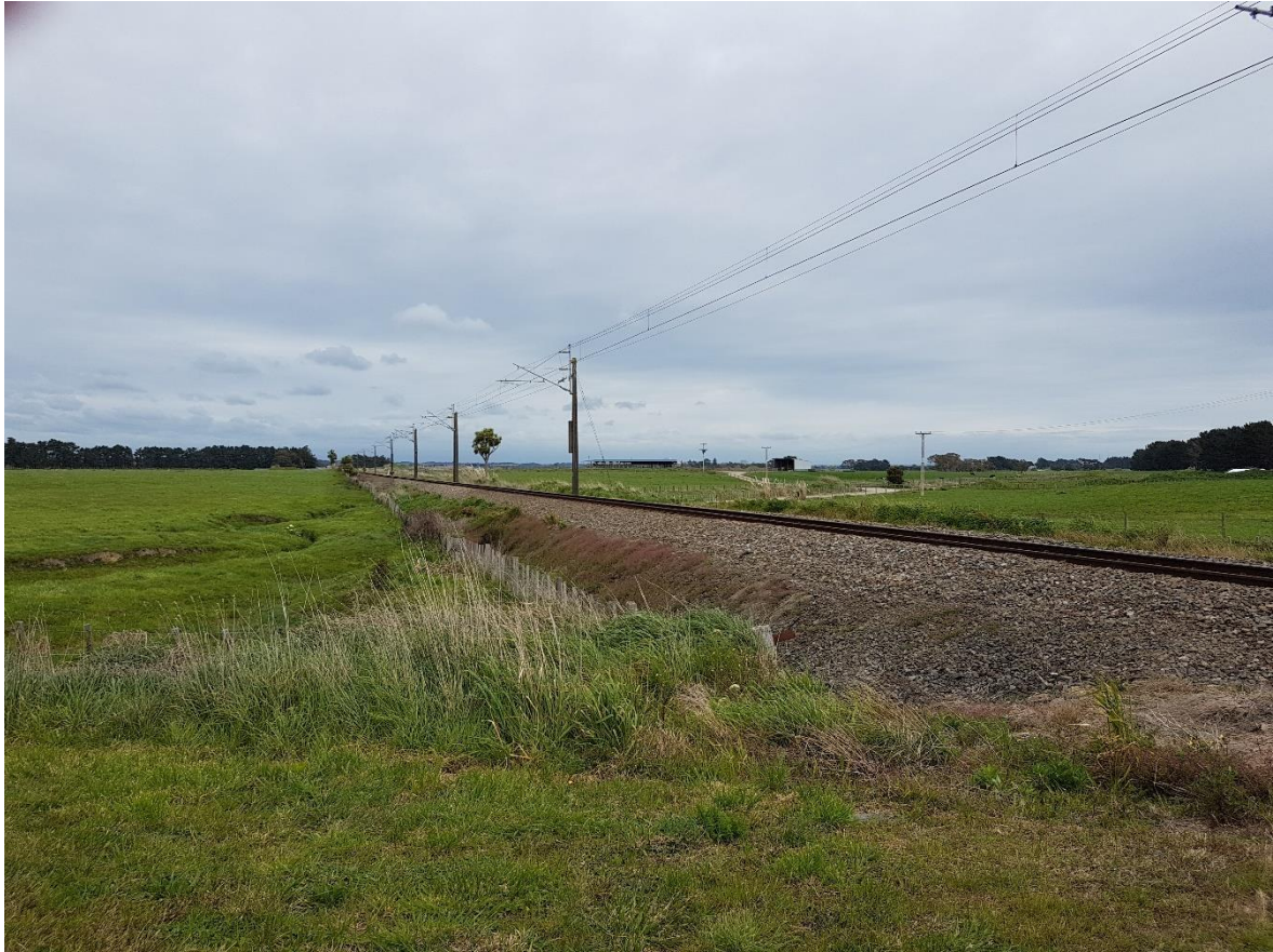
Figure 5: East Approach – looking south from 1.5m back from limit line
