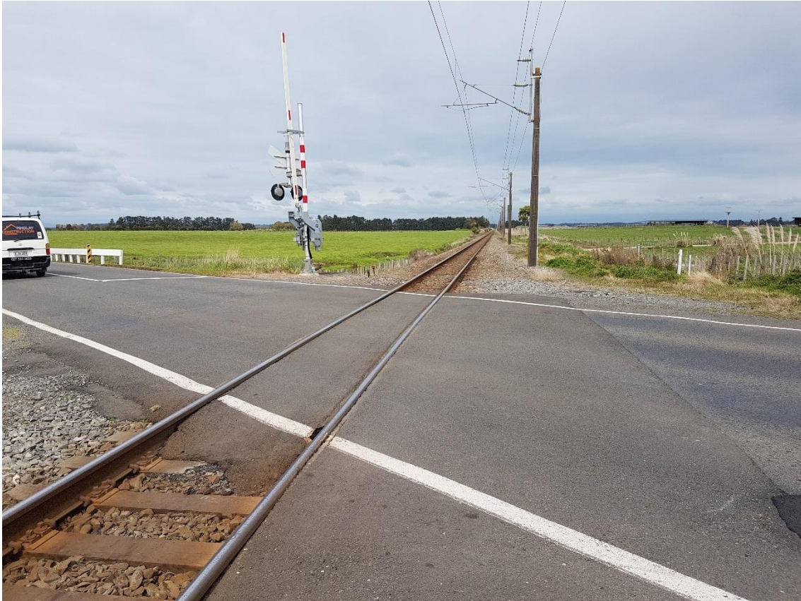
Figure 9: Panel Condition and approach surfacing
