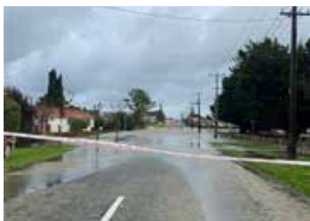
Flooding 21 May 2023 - Marumaru Street, Marton.
