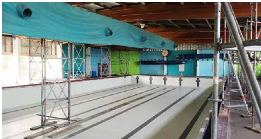
Bracing inside the Marton Swim Centre.
