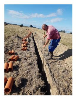
4. Photograph 4 shows the joint area of the tile systems where they flow into the drain. That stretch of tiles is laid through the low points of the land and all joins together to a main tile.
