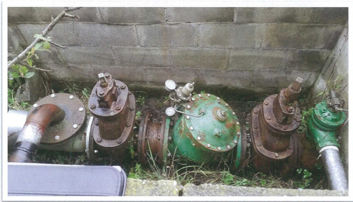
Condition of existing valves and PRV
