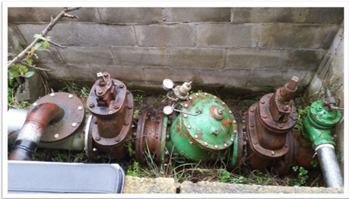
Condition of existing valves and PRV
