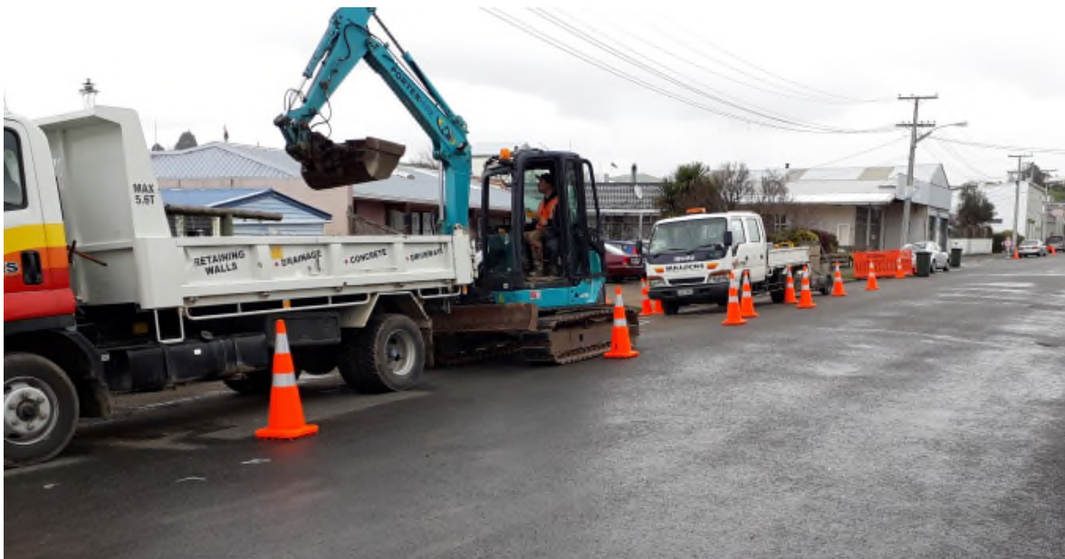
B Bullock crew installing water main at Tui Street
