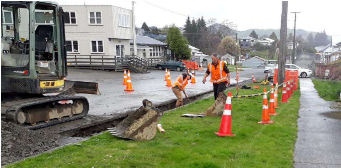
B Bullock crew installing water main at Toroa Street
