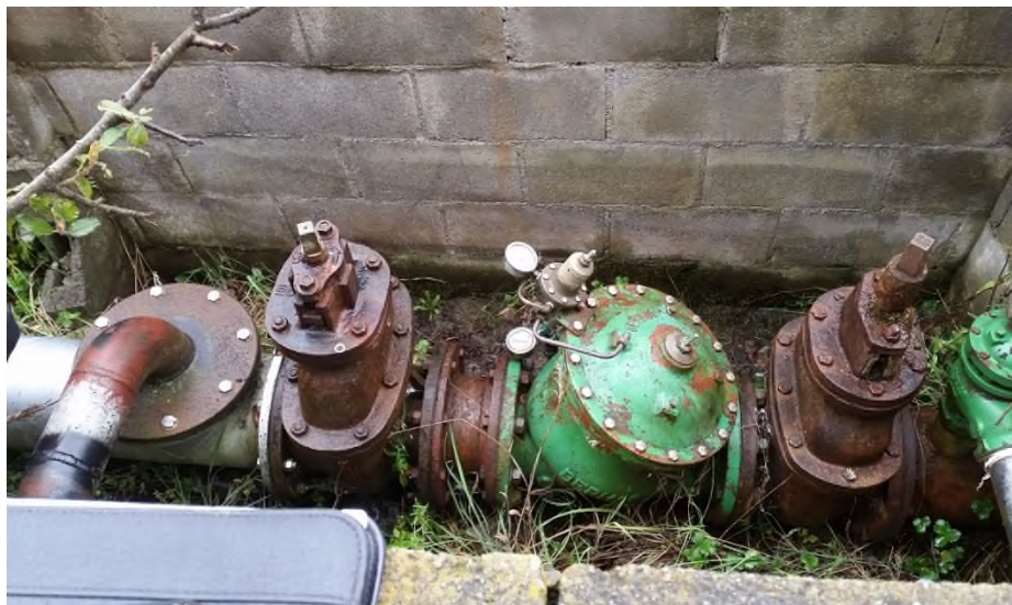
Condition of existing valves and PRV
