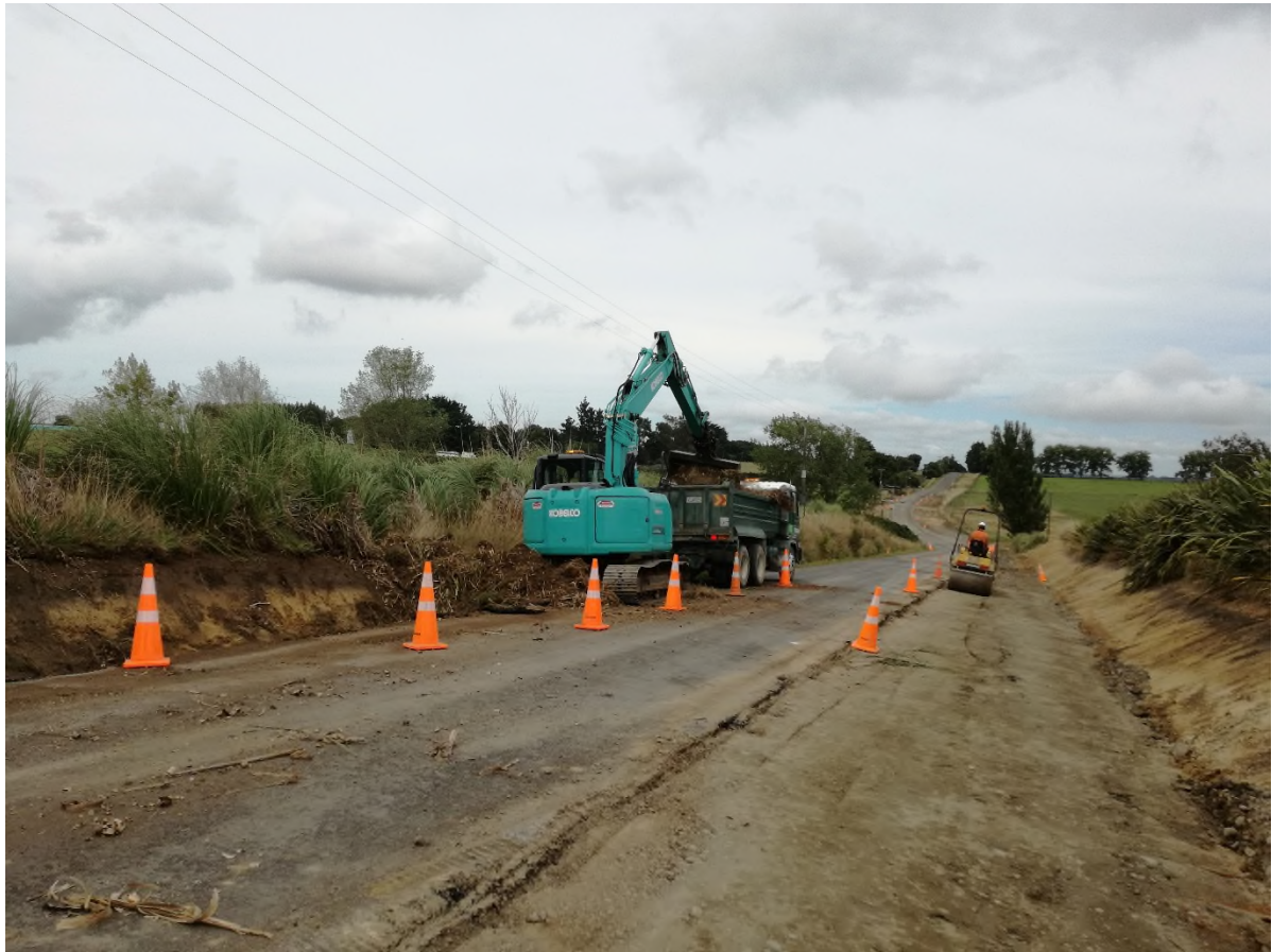
Photo: construction of the safety shoulders in preparation for the pavement overlay
