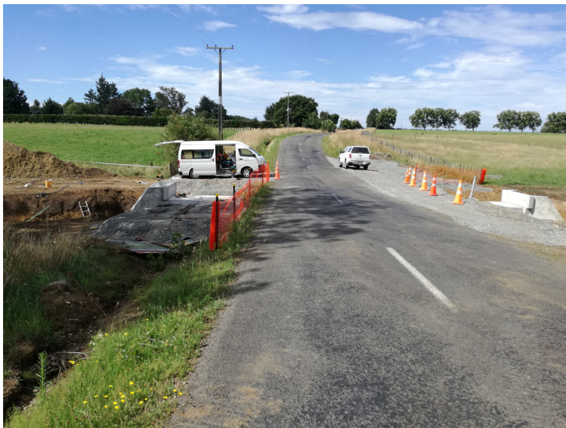
Photo: extending the box culvert in preparation for construction of the safety shoulders and pavement overlay
