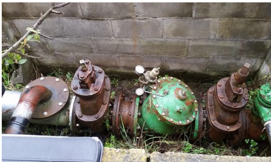
Condition of existing valves and PRV
