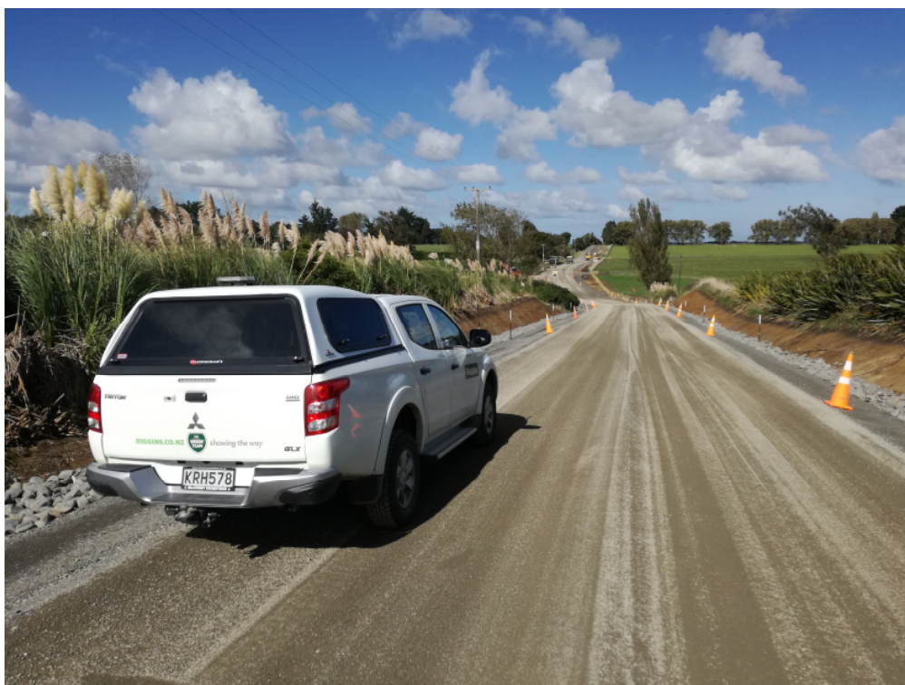
Photo: Galpins Road - final preparation prior to first coat sealing
