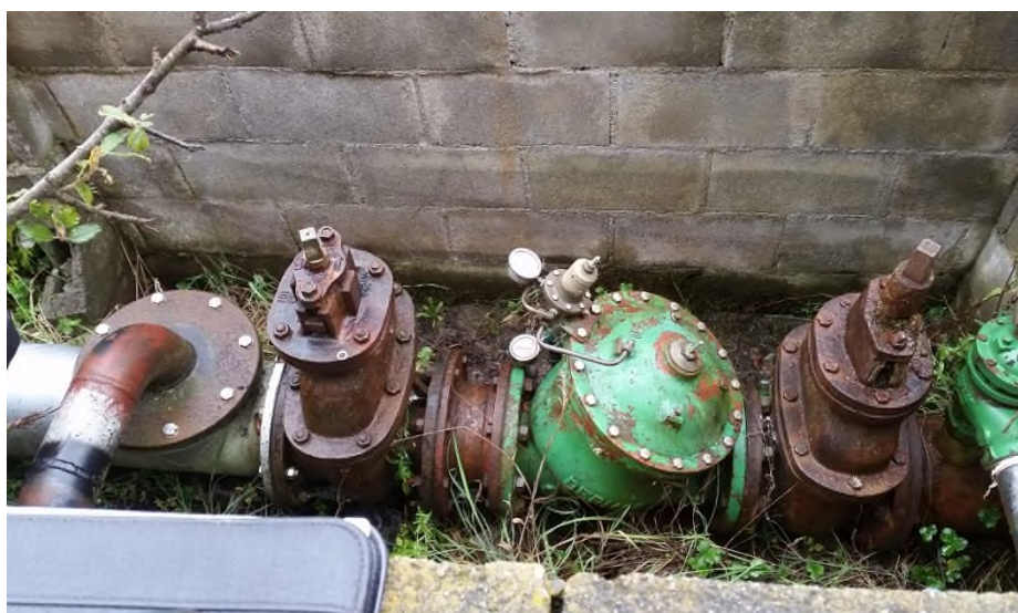
Condition of existing valves and PRV
