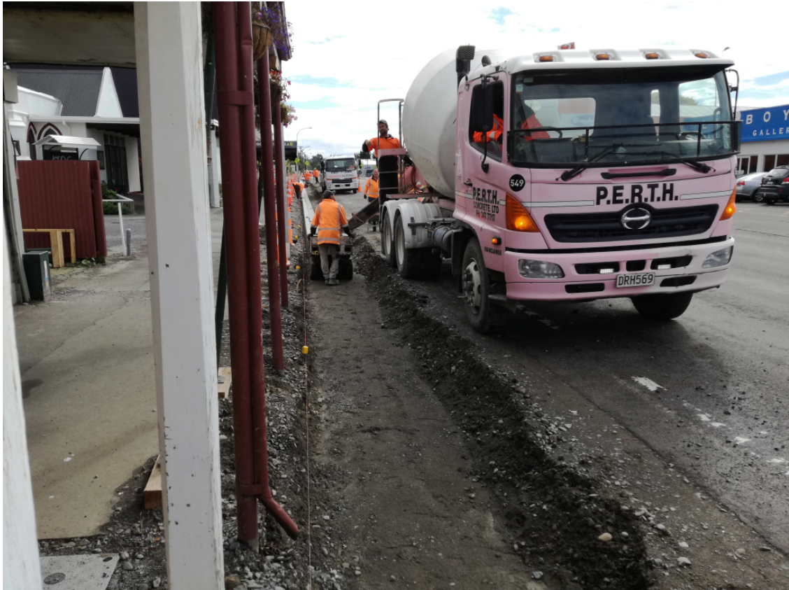
Photo: Broadway – pouring kerb and channel
