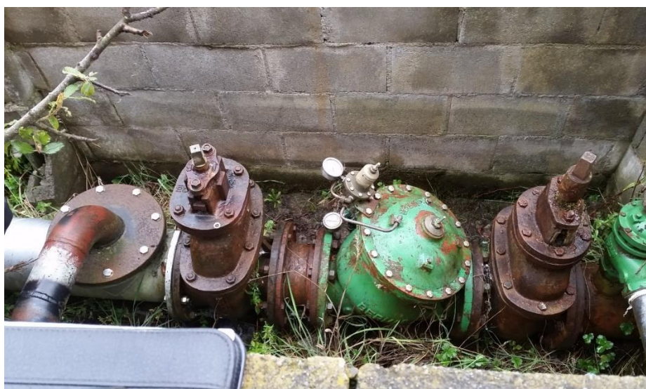
Condition of existing valves and PRV
