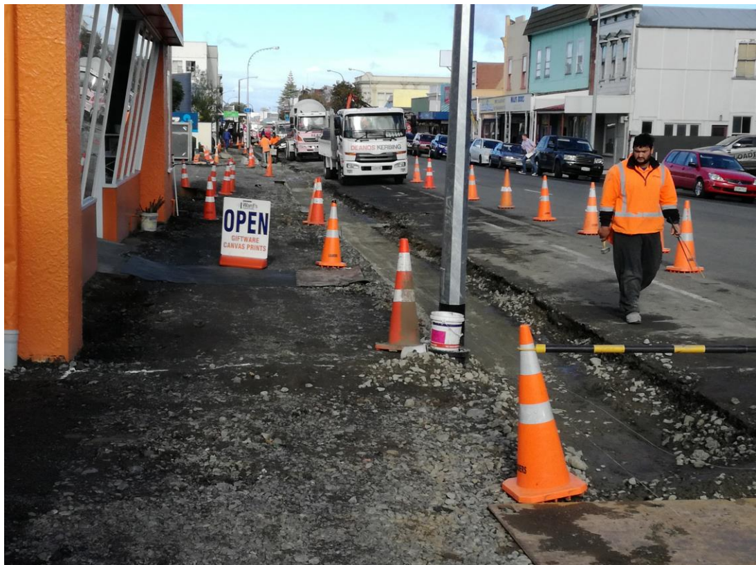
Photo: Broadway – pouring kerb and channel outside Wards Furniture
