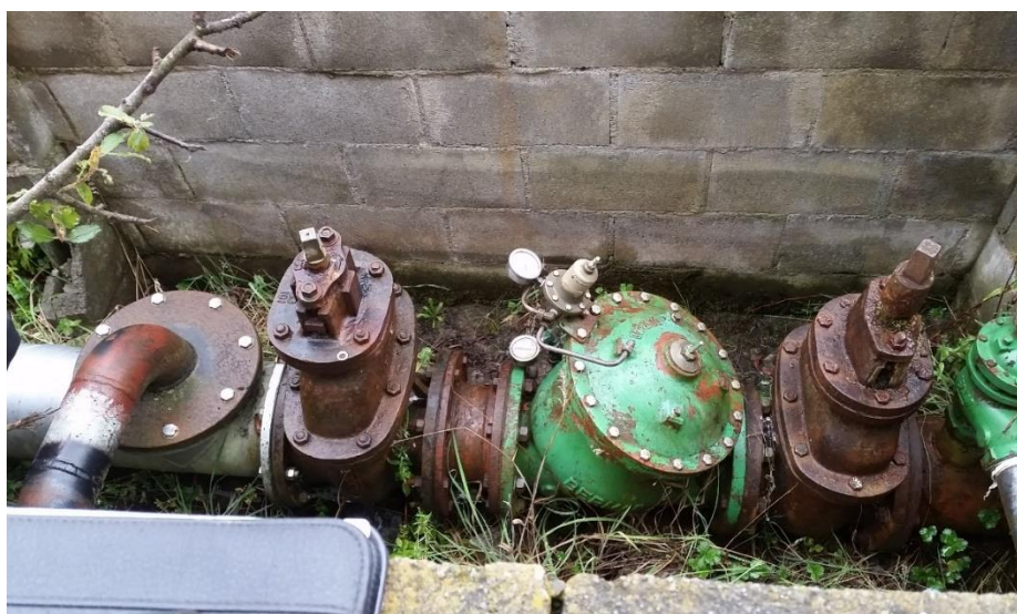
Condition of existing valves and PRV
