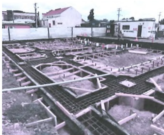
Ground beams & HD Bolts
