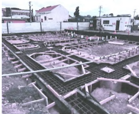
Ground beams & HD Bolts
