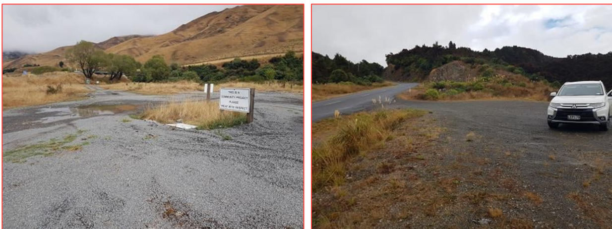
Figure 5-1: Rest Area – Springvale Suspension Bridge (Left) and the Kaweka Range (Right)
