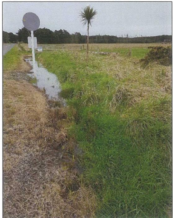
Photo 4: Overgrown Roadside Drain
