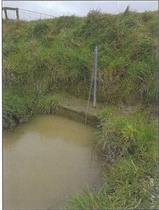
Photo 8: Drain Blocked by Flap Valve (Town Side)
