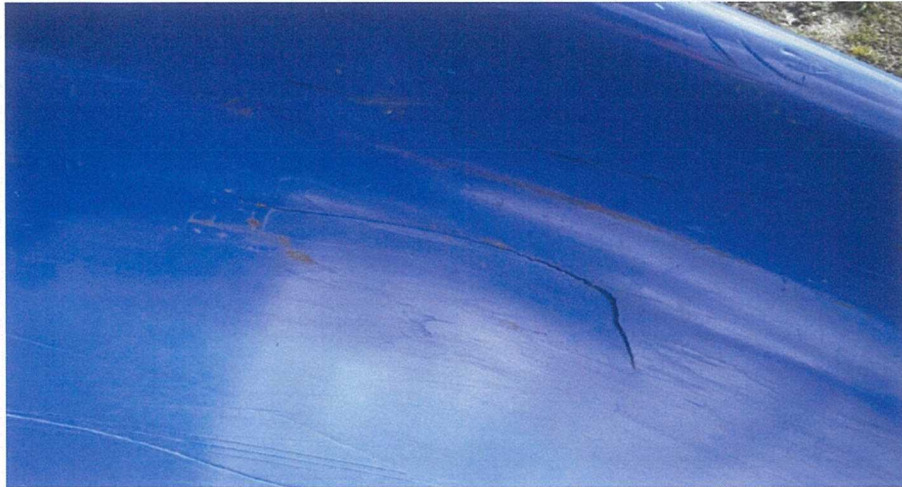
Photo 2 –Cubby roof damage
