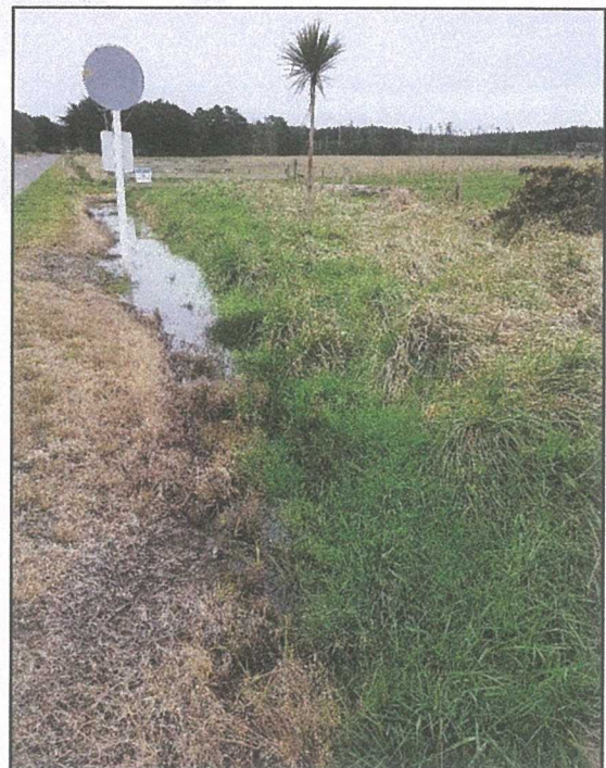
Photo 4: Overgrown Roadside Drain
