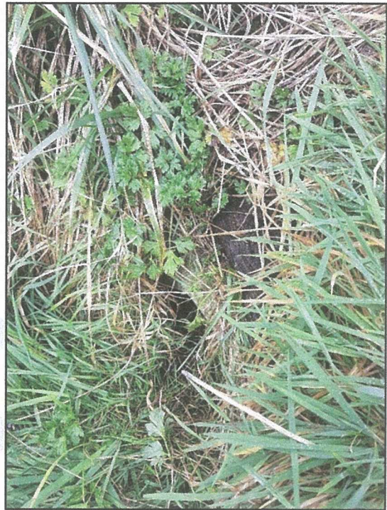
Photo 4: Overgrown Roadside Drain
