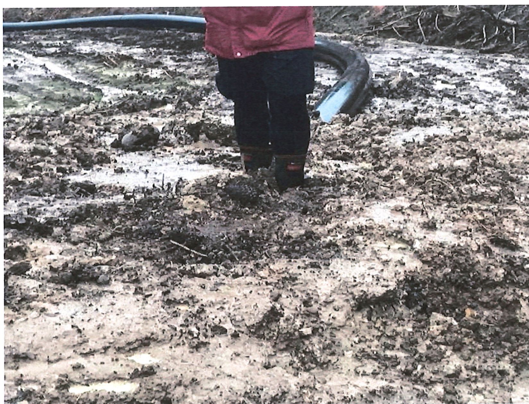
Unconsolidated and uncontrolled sediment flows adjacent to dam spillway and Tutaenui Stream
