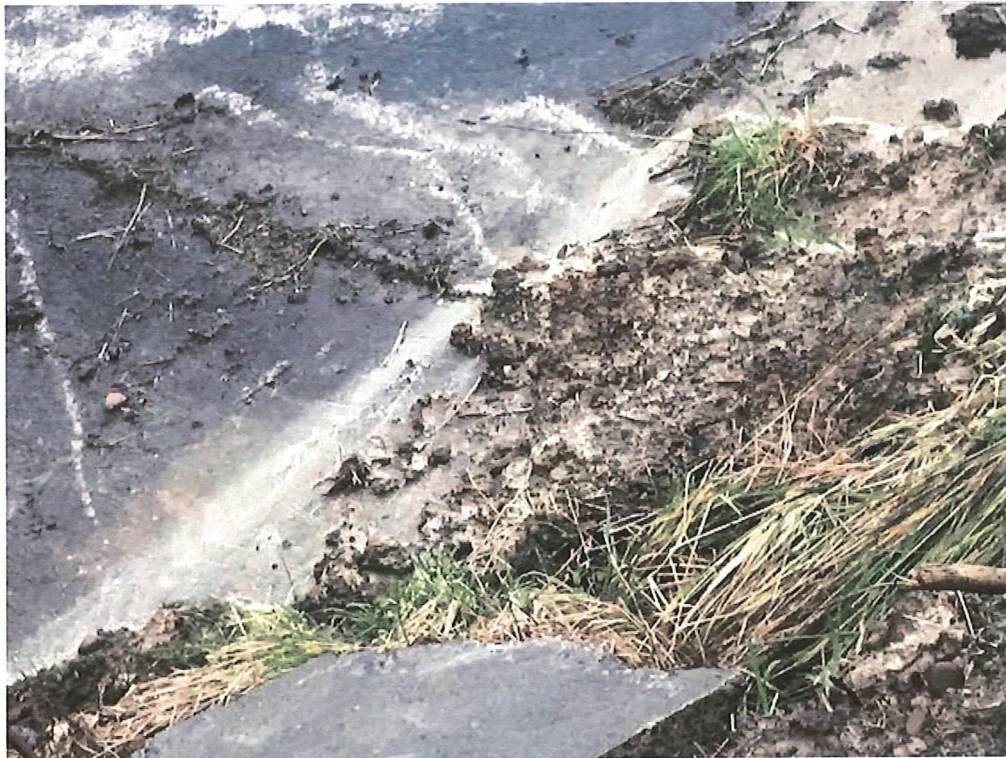
Dumping of waste material into dam spillway
