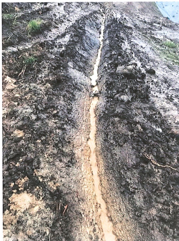
Deliberate diversion of uncontrolled overland flow through construction site to the Tutaenui Stream
