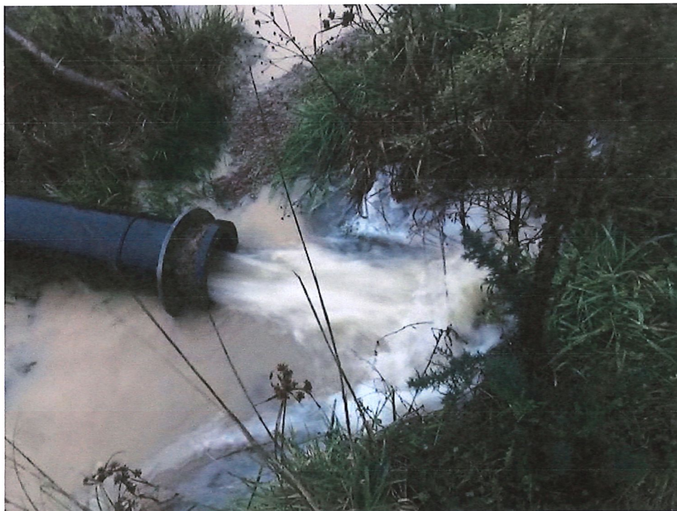
Discharge of sediment-laden stormwater into the bed of the Tutaenui Stream
