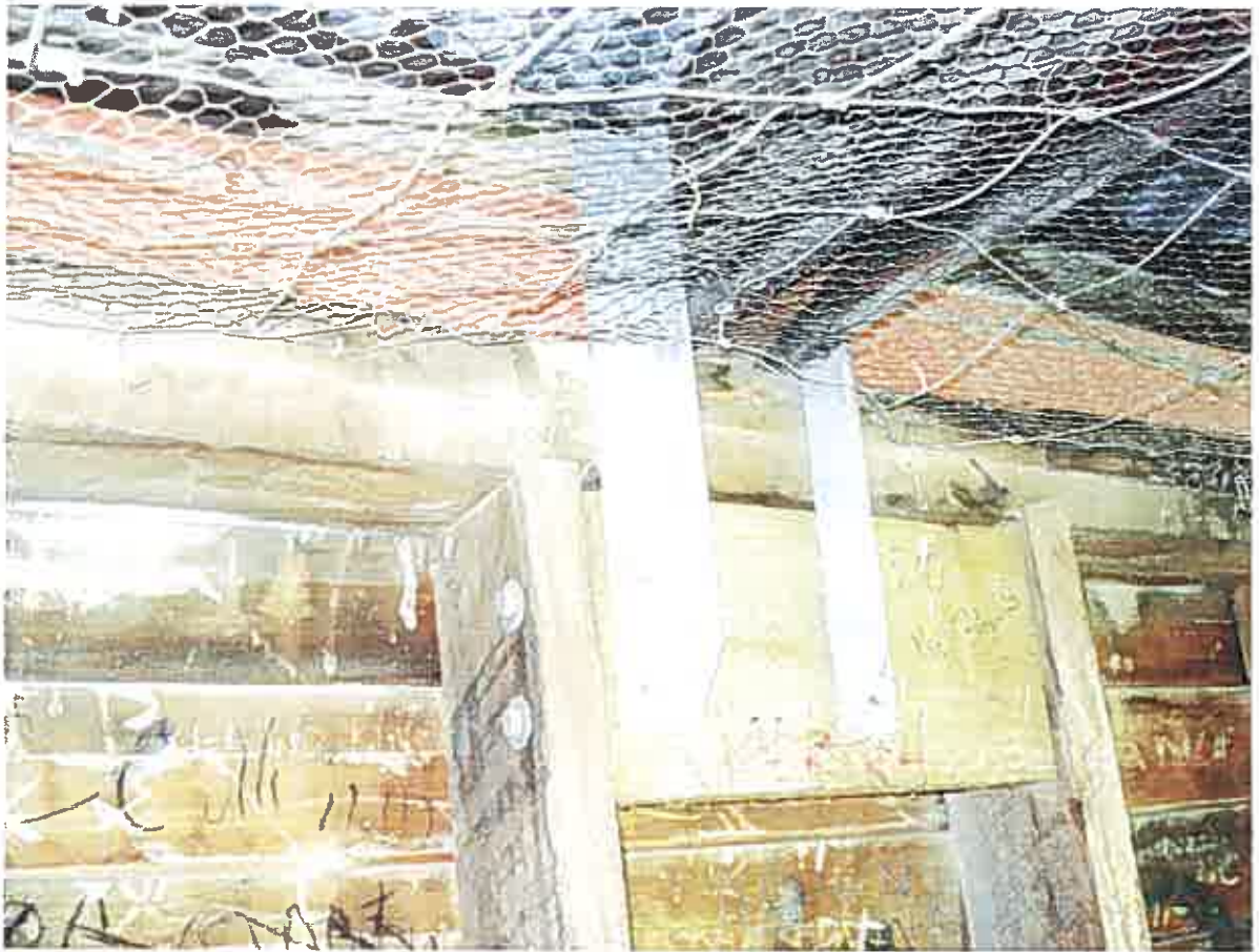
Photo 9 – Roof Truss Additional Fixing
