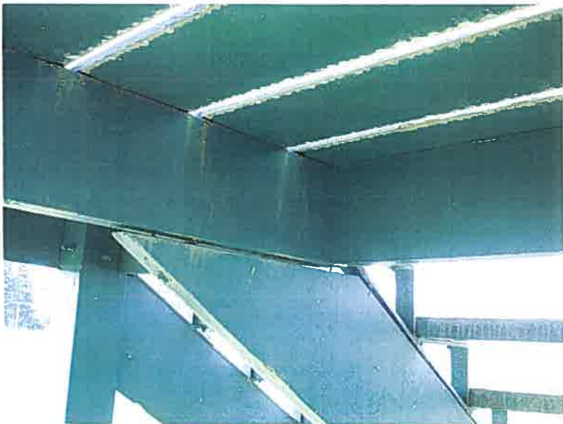
Photo 6 – Stair Stringer Connection
