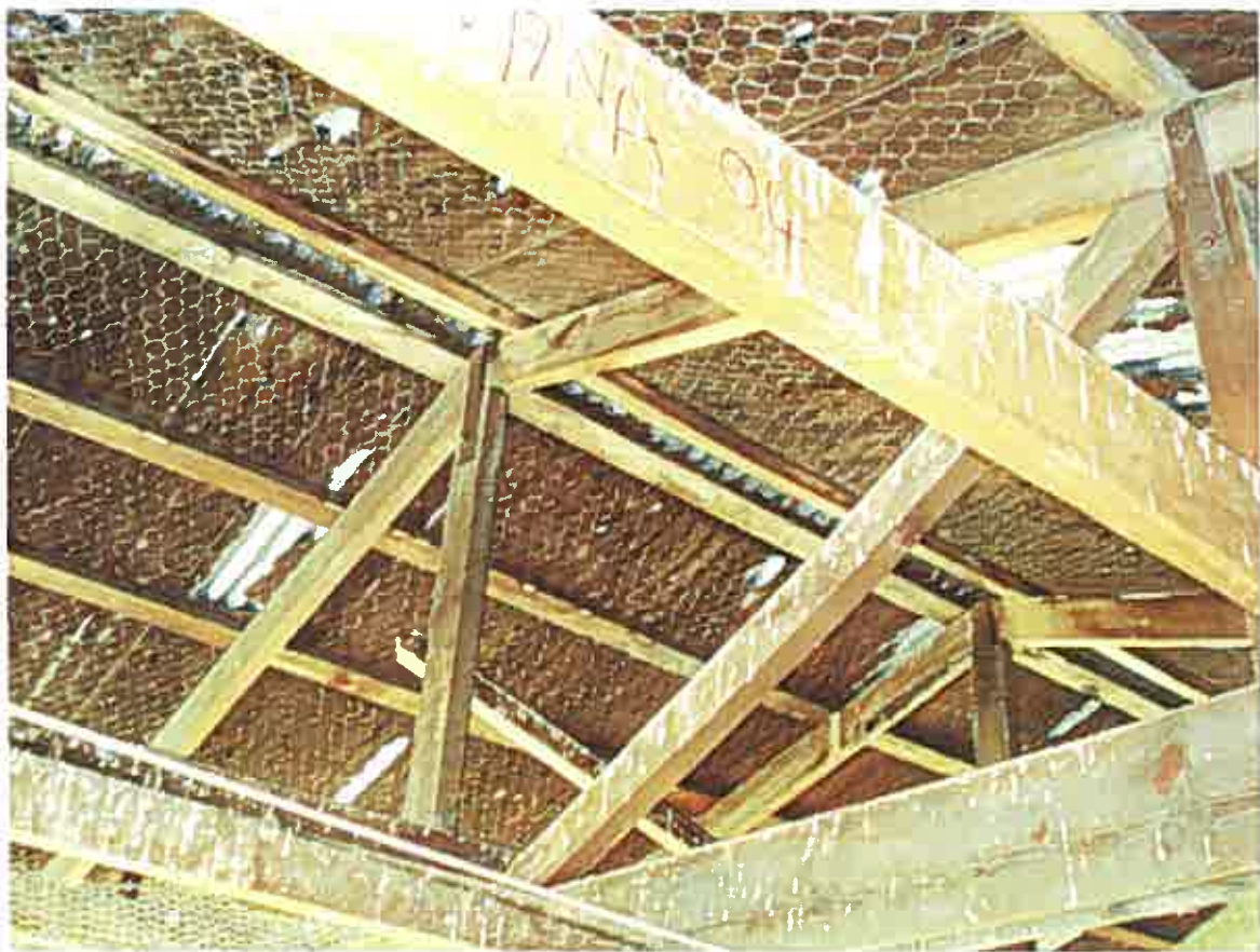
Photo 8 – Roof Truss
