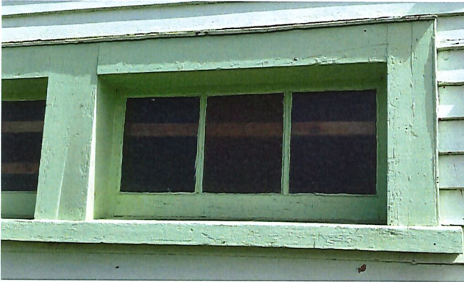
Typical existing window jammed in closed position
