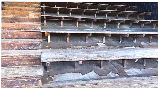
Damaged waterproofing under seating
