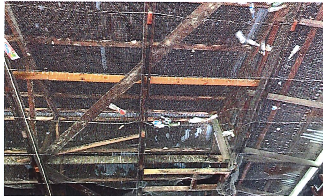
Condition of roof above seating
