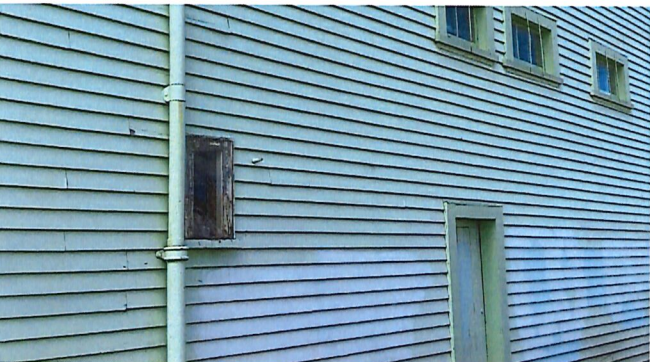
Original weatherboard cladding
