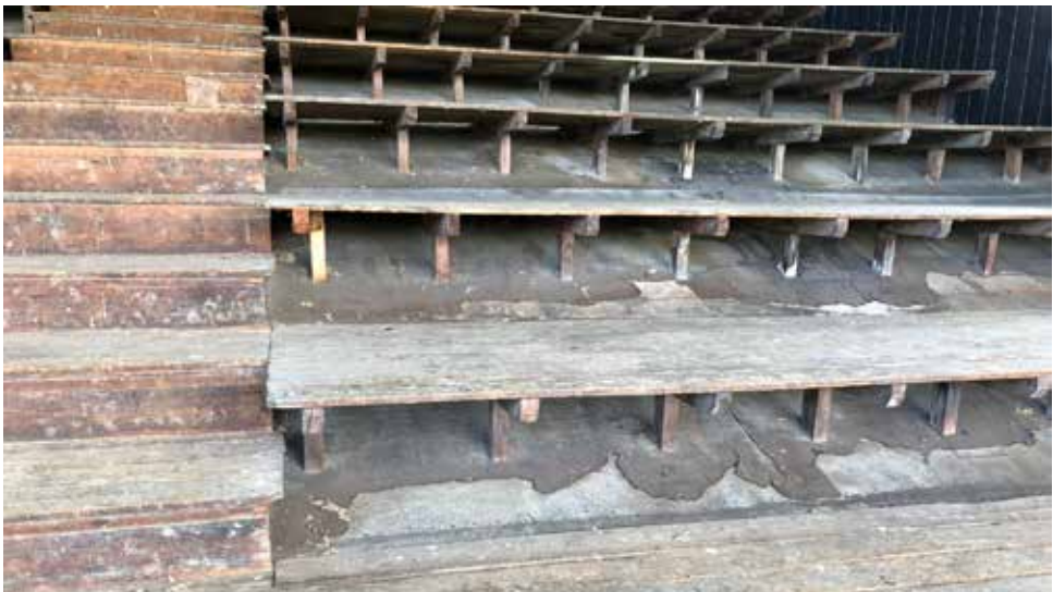
Damaged waterproofing under seating
