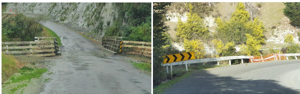
Figure 11: Non-complying barrier systems examples. Left – one-lane bridge with timber sight rails (requiring cleaning), steel tube bridge rails and no approach terminal treatment (Turakina Valley Road); right – sight rail above steep ravine subject to recent crash damage (Kawhatau Valley Road).
