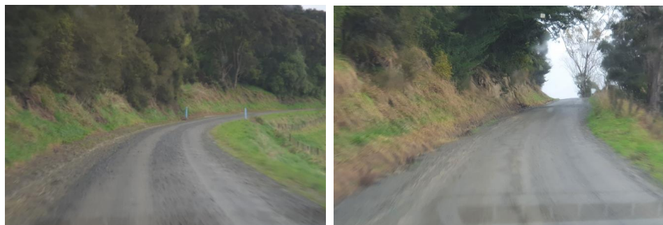
Figure 6: Unsealed road examples (Turakina Valley Road). Left – effective left-hand table drain, good surface shape and materials, well maintained culvert markers, but requiring right-hand high shoulder removal; right – inadequate left-hand table drain capacity resulting table drain scour during high rainfall, high shoulder (right-hand side) and vegetation encroaching into clearance envelope.
