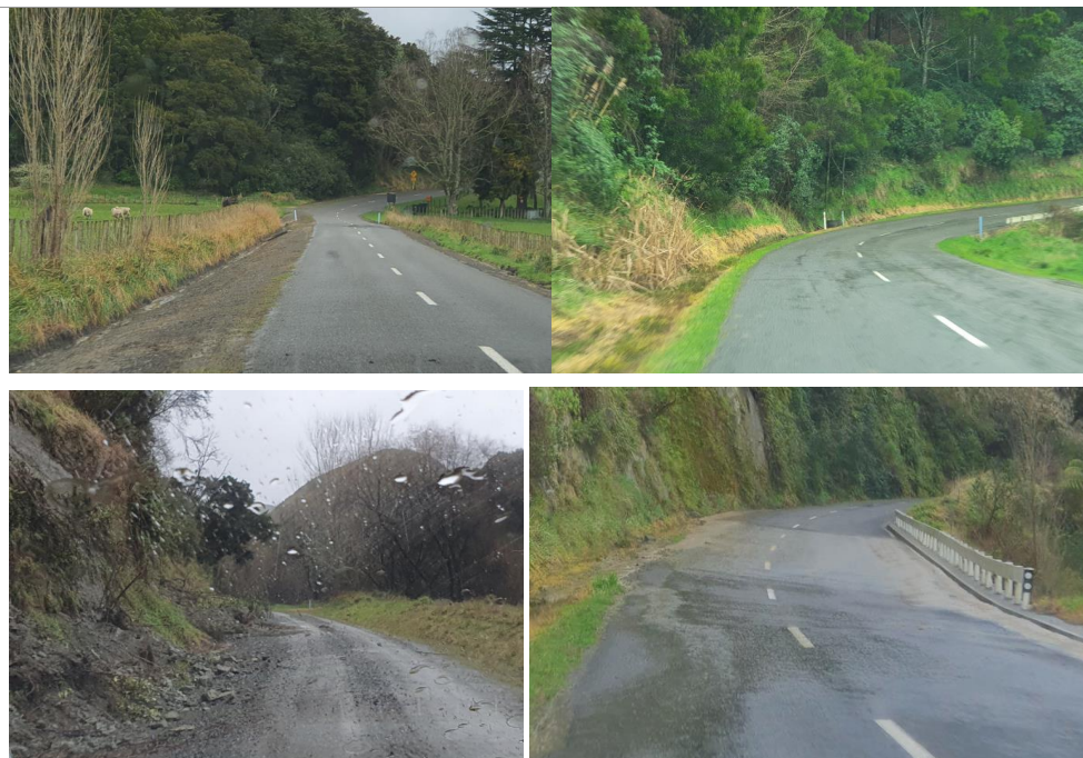
Figure 1: Examples of good drainage and drainage improvement opportunities (Turakina Valley Road). Top left – effective road berm and table drain intervention completed as part of pre-reseal repairs; top right – ineffective table drain in low-lying area requiring clearing to reduce risk of pavement saturation / premature; bottom left – small slips / cut batter fretting blocking table drain; bottom right – inadequate table drain capacity resulting in water sheeting across the road affecting motorist safety and likely cause of historical emergency reinstatement treatment on the opposing roadside.
