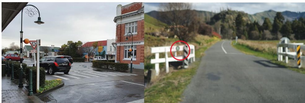
Figure 13: Pedestrian and cycling safety improvement examples. Left – pedestrian priority (zebra) crossing requiring ground surface indicator pavers and belisha beacon poles requiring remarking of bands; right - existing less conspicuous cycle trail signage (Kawhatau Valley Road).
