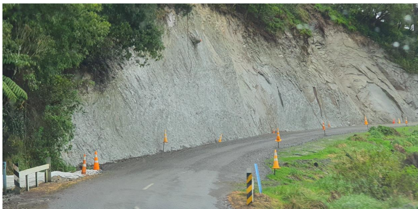
Figure 14: Use of waratah standards to support TTM cones, thereby introducing a new roadside hazard (Turakina Valley Road).
