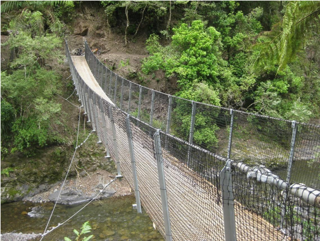
Typical swingbridge with timber deck similar to that recommended (Motu Trail)
