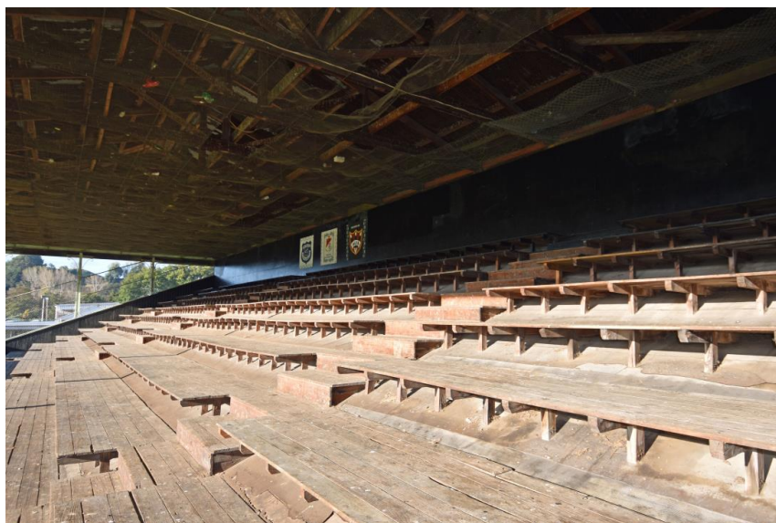
Figure 2: Looking across grandstand to the south-east, showing detail of the benched seating and exposed roof trusses above, Joanna Barnes-Wylie, Heritage New Zealand Pouhere Taonga, 29 April 2022
