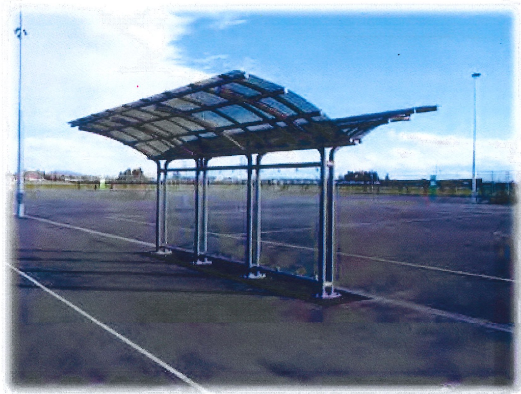
Recently installed shelters provide spectator protection from the elements
