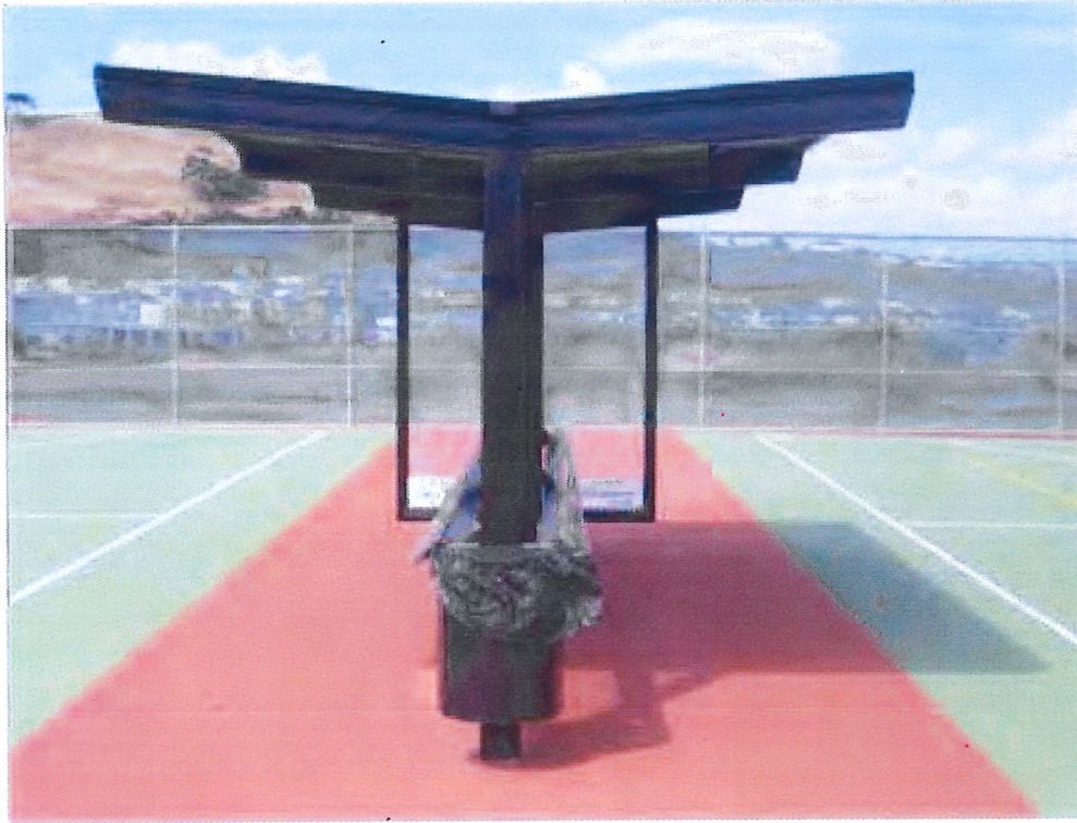
Photo 5: Courtside Shelters, Side View
