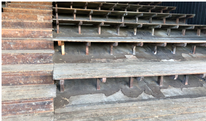
Damaged waterproofing under seating
