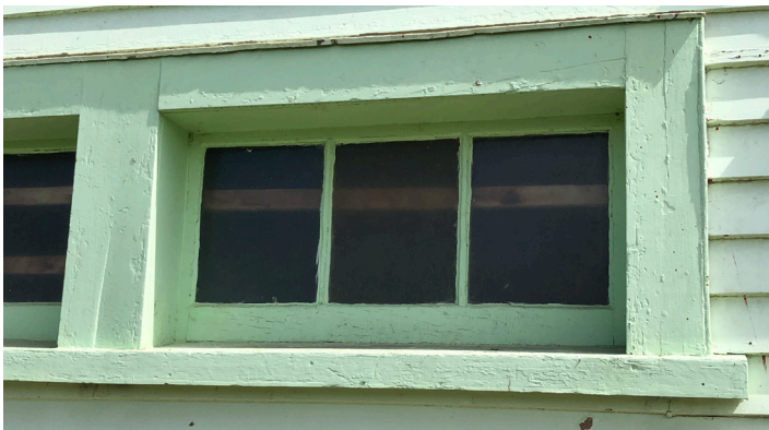
Typical existing window jammed in closed position
