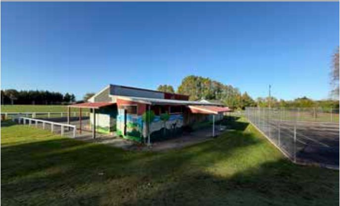
Kitchen and shaded structure facing the netball and tennis courts.
