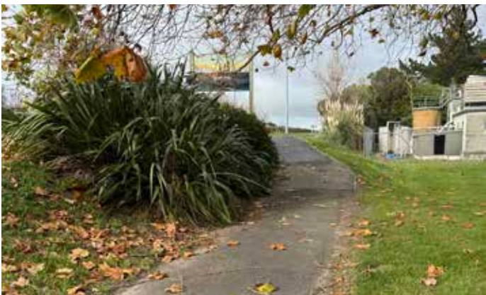
Cycleway access to bridge.
