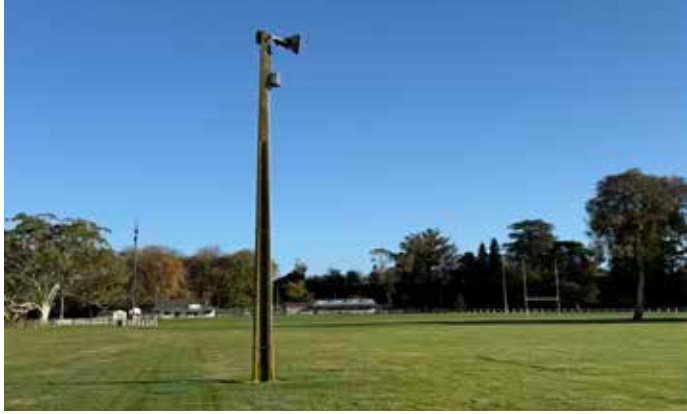
Sports field lighting.
