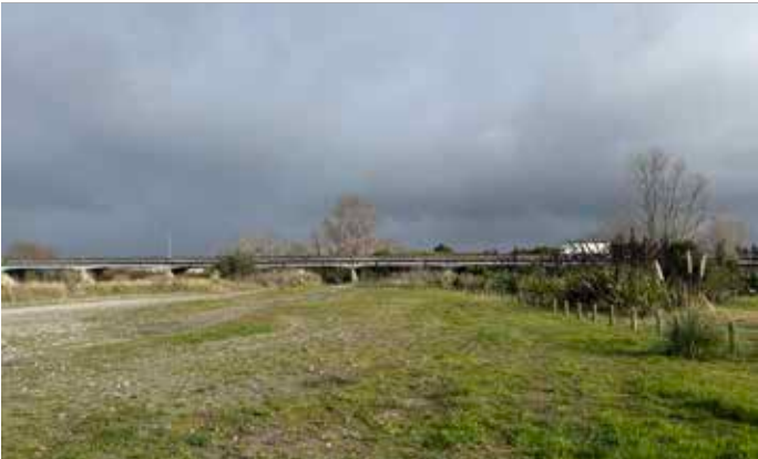
Car parking area.
