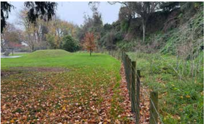
Fenced creek area at the back of playground that sometimes overflows and floods the playground.
