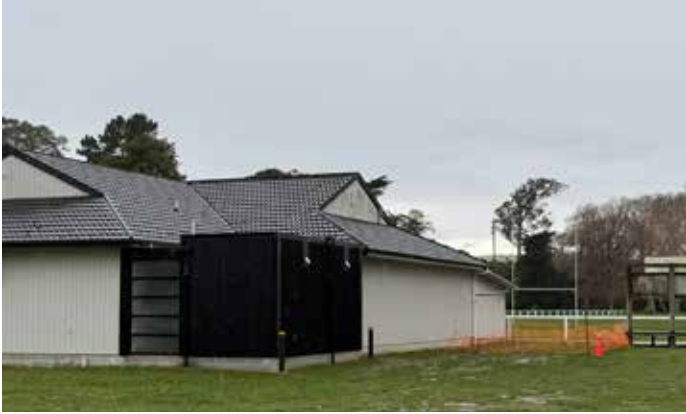
Rugby clubrooms with space to expand to the right of the photo.
