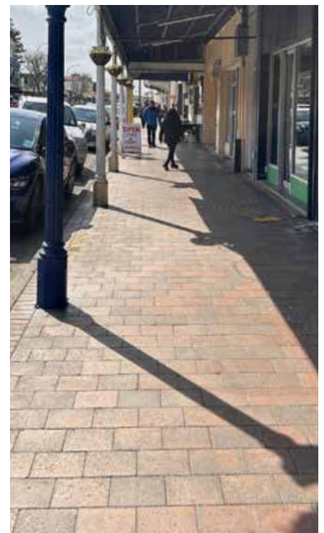
Existing concrete paving blocks in Marton town centre are discoloured and worn smooth.
