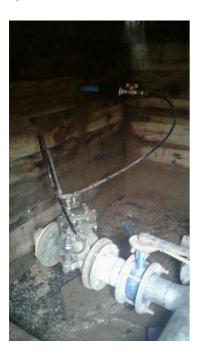
This valve is leaking and needs to be re-kitted. The valve was also leaking from the indicator assembly "O" rings which need to be replaced at the same time.
