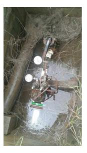
This valve was completely submerged in the pit, a brass fitting had cracked and was filling the pit. This fitting was replaced on the spot. Unfortunately, due to a lack of system demand, other than a hydrostatic test, this valve was not able to be function tested.
