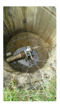
This direct acting pressure reducing valve, and the associated Bermad 730.050Q quick relief valve, were both working perfectly.
