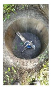
This valve is an irrigation spec Bermad PRV. It is not the correct valve for this application, a Wilkins NR3040 and up/downstream gauge on tees would be the best choice.
