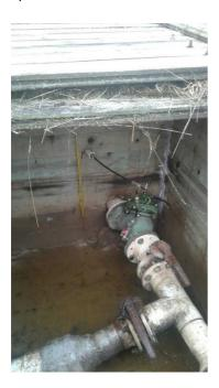
This valve tests out ok, but when convenient it would be useful to fit a ball valve where the line goes into the wall to allow easy access to test.
