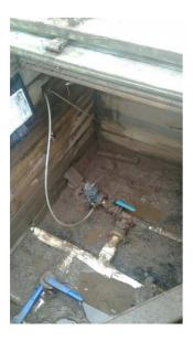
This valve appeared to be sound, however the #66 float pilot was not working properly. This float pilot may have lost its "timing" (the barrel had been rotated putting the ports out of sequence).
