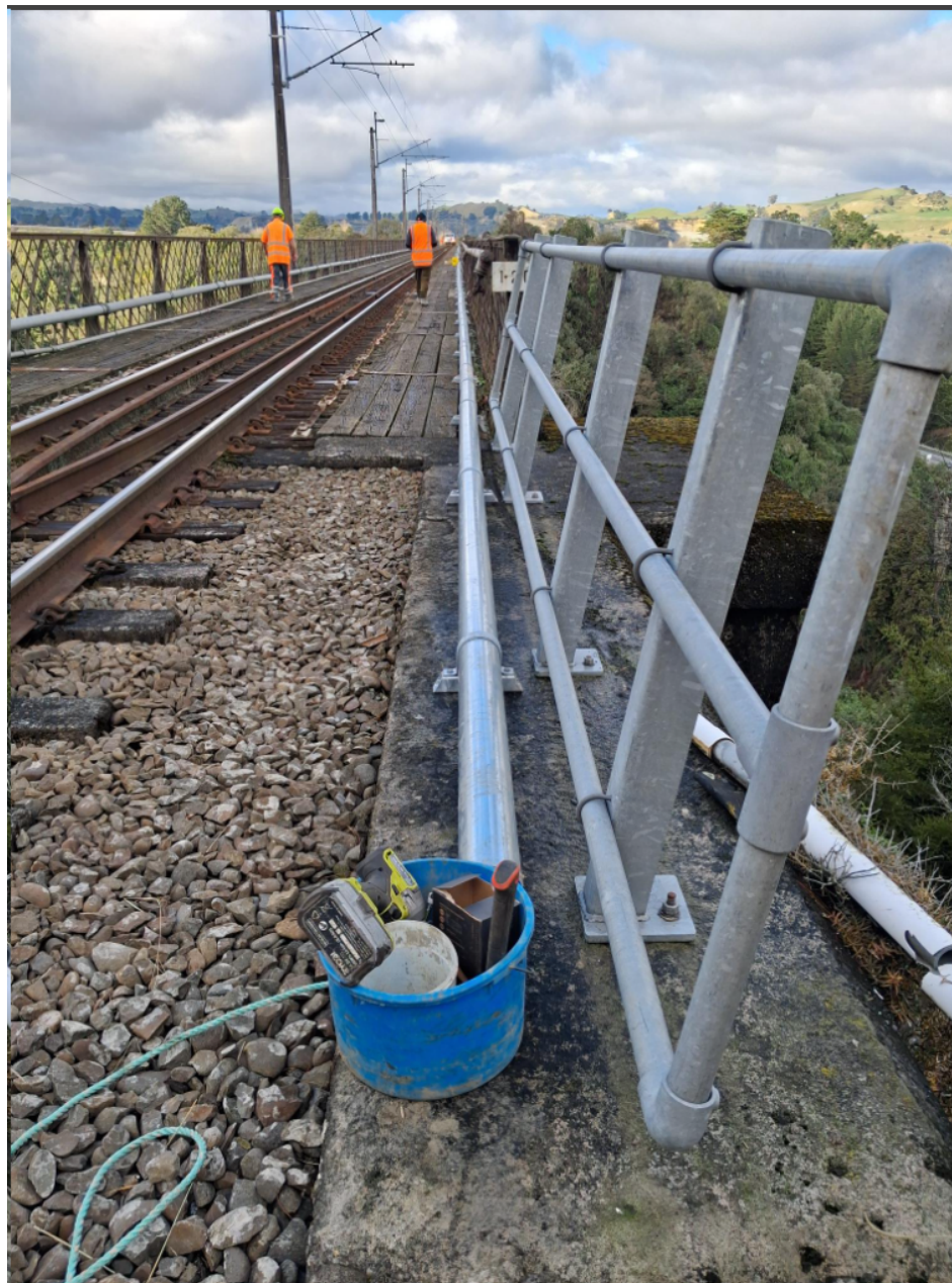
Appendix 2 - Makohine Viaduct Photos
