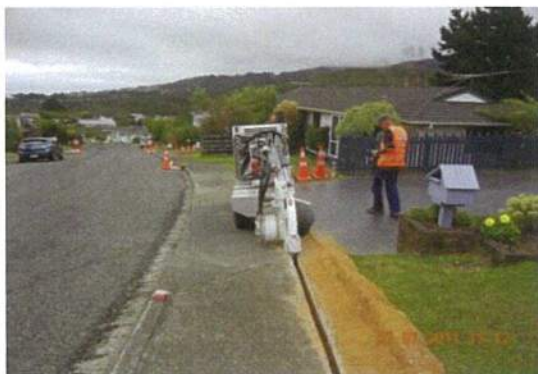
Duct and cable installation
