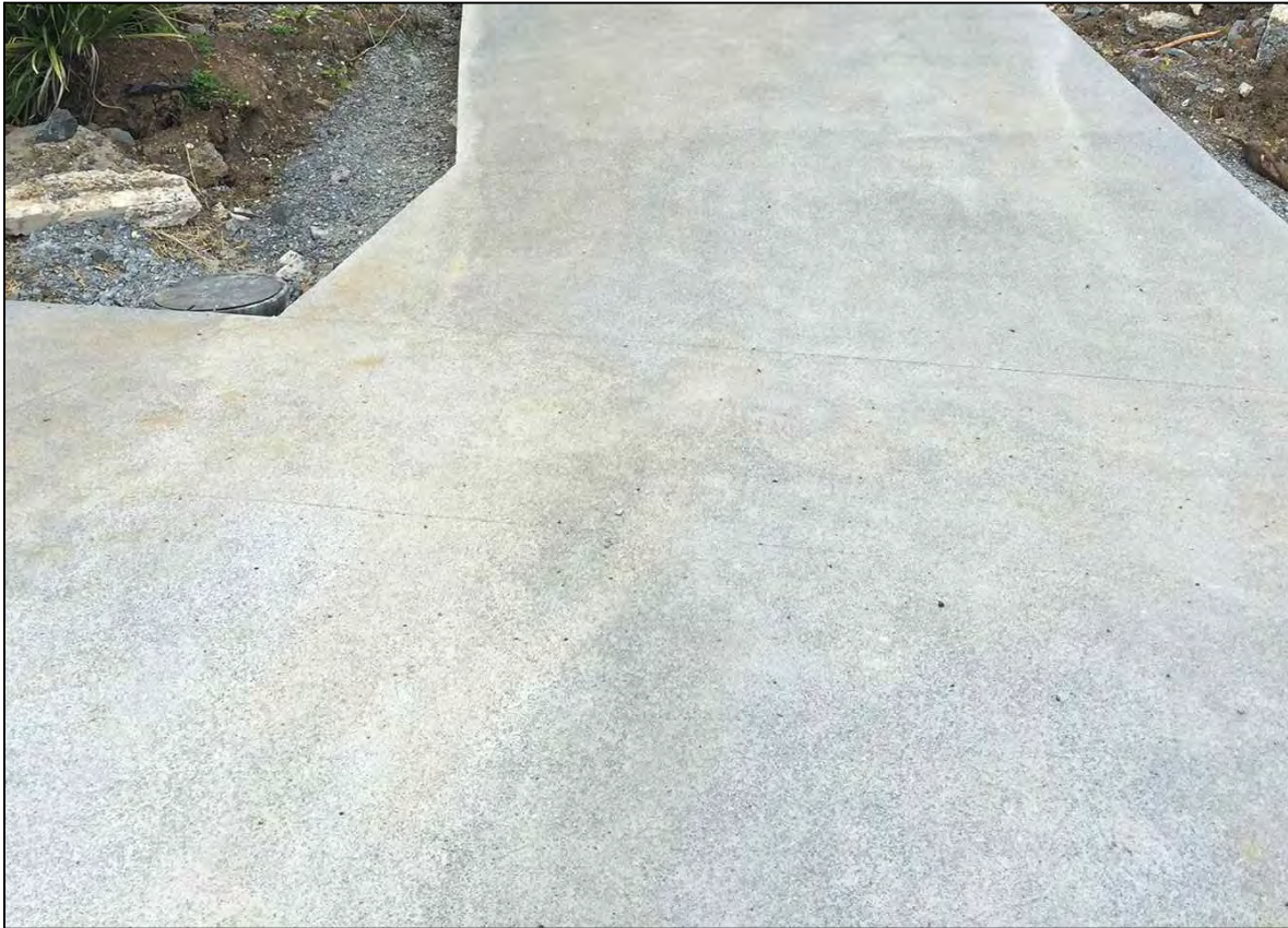
FOOT PATHS 100mm Thick Concrete footpaths.
