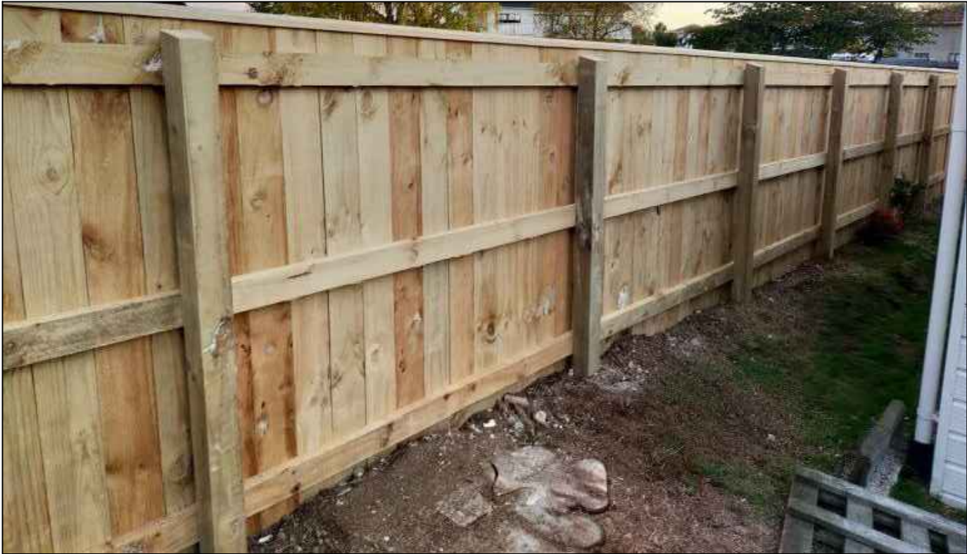
FENCING New Standard 2.0m high Timber Fencing. 300 wide concrete mowing strip under.
